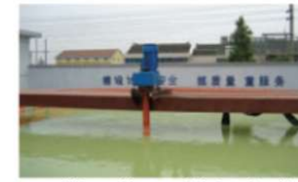
Mixer without prefabricated walkway
